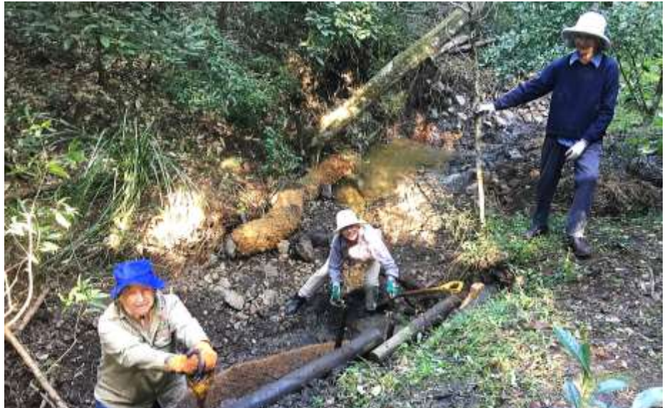
Florence, Susan and Nancy building the 'Girlin Wall' - part of our creek erosion control
